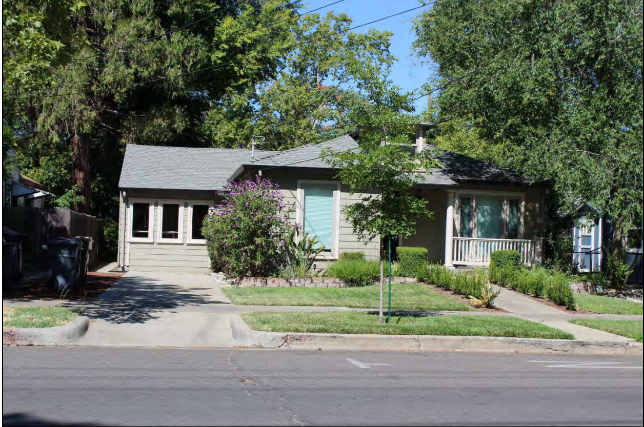
Photo 1 of 15: Front (east) façade, looking west
