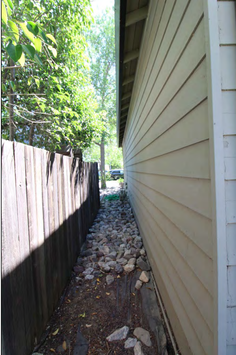
Photo 5 of 15: North side façade, looking east
