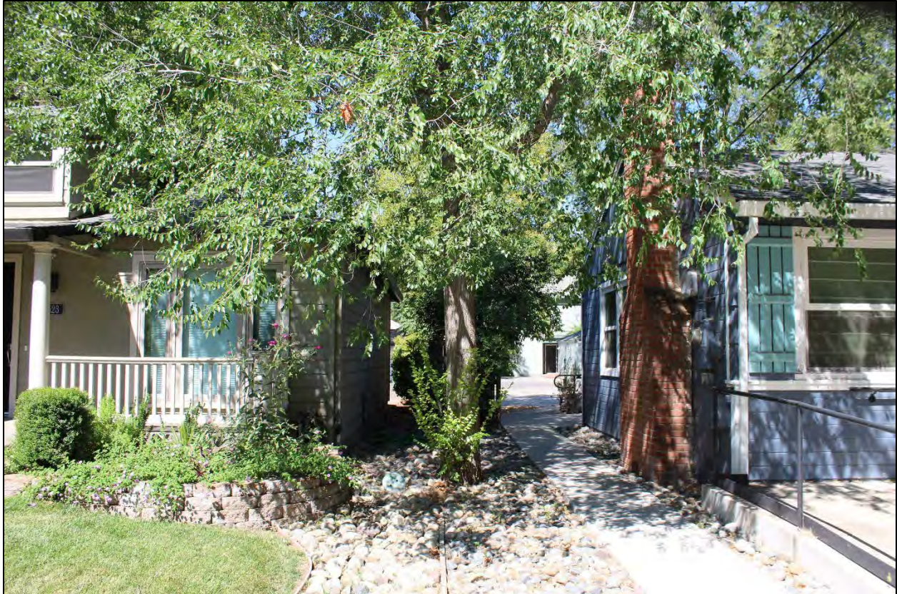
Photo 6 of 15: North side façade, looking west
